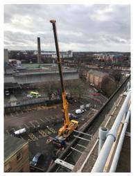
Whilst the internal work is starting to take shape, work has started to ensure the building is fully equipped to support the new clinical areas. New air handling units have been placed on the roof. In order to do this two crane lifts were needed, one to put down the steelwork to support the air handling units and the second to lift the units into place. Crane lifts are dependent on weather conditions. Fortunately, the lifts were able to go ahead as planned.
